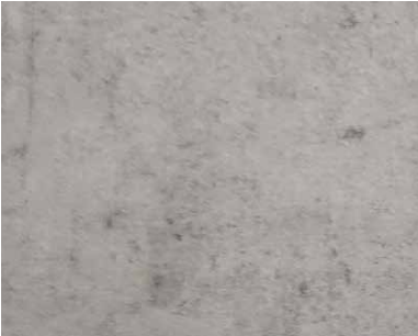
MACK AVE CONCRETE
